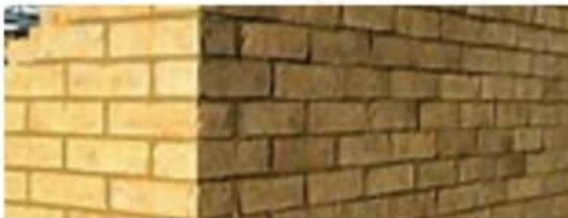
Figure 7.1: Bricks bonded using mortar to form a wall
